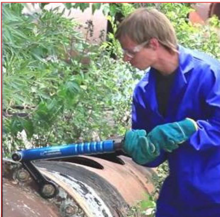
*BMG's new Slogging Hammer is used to loosen and tighten bolts and nuts quickly and easily.*
